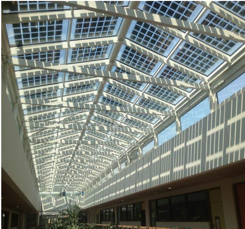
Figure 18: Canopy with transparency achieved by alternating classical c-Si PV-cells.
